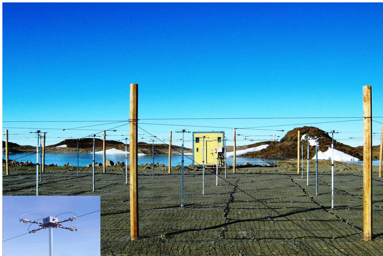
Fig. 16: South-east view of the installed imaging Riometer at Maitri. It includes the antenna and the hut (yellow color hut) where the receiver unit is kept
